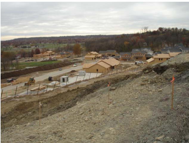
Cheyenne Village Construction
